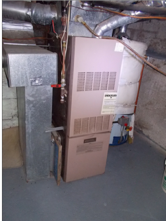
Photograph 8 - View of the furnace and water heater.
