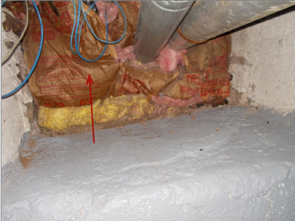
Photograph 10 - View of the fiberglass backing in the basement, Sample 10.
