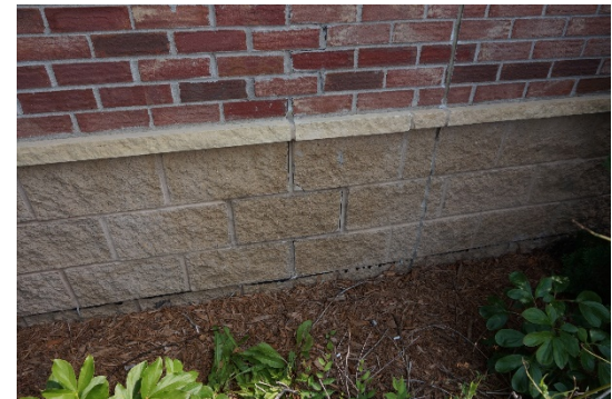
Cracking brick and CMU on west side
