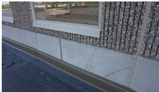
Cracked precast walls
