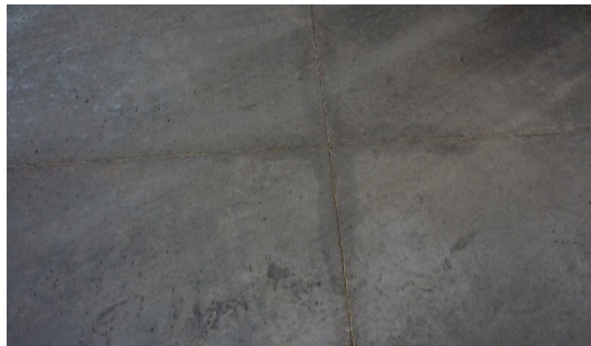
Mild salt corrosion at slab joints of PW Garage
