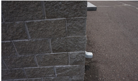
CMU degradation on northwest corner
