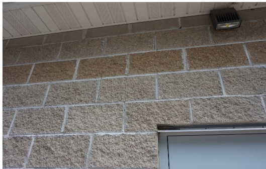
No lintels on west doors (B)
