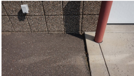
Bituminous settling near stoops
