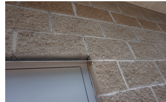
No lintels on west doors (C)
