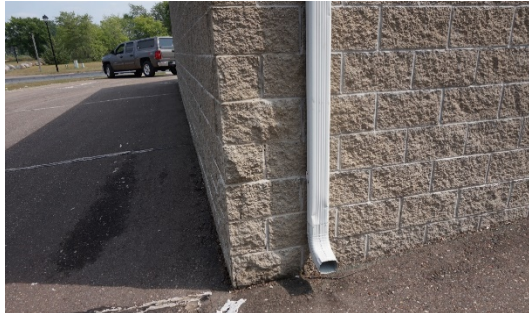
CMU degradation on northwest corner
