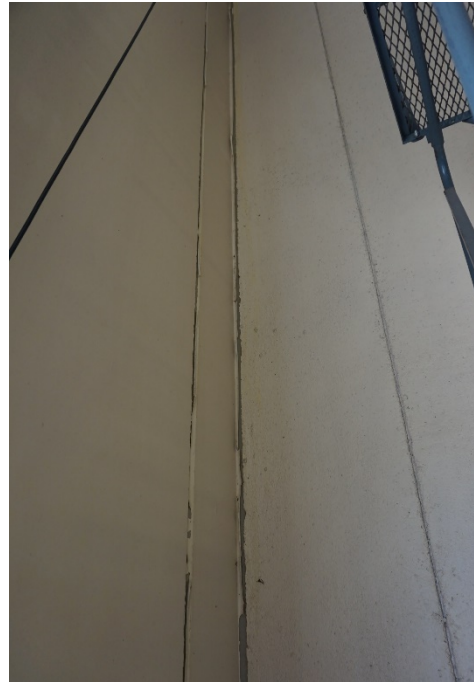
Paint deteriorating at wash bay
