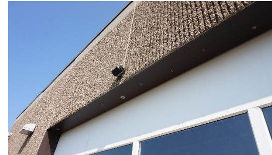
Water leaking through OH door lintel screws
