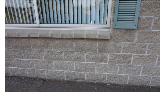
CMU cracked under east window
