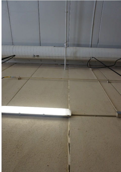
Sealant pulling away at Wash Bay PC joints
