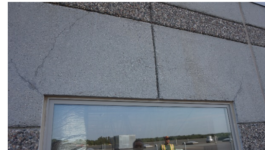
Cracked precast walls
